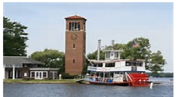
Clock Tower & Pier Building
